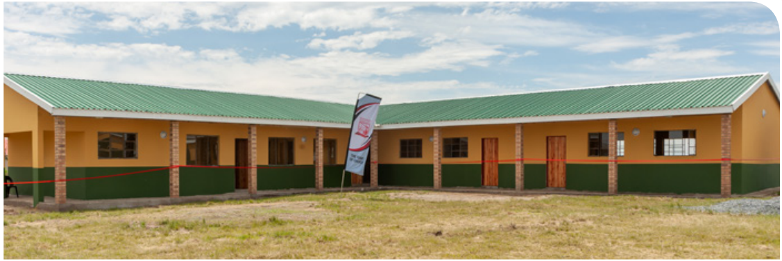
Image of the completed school
