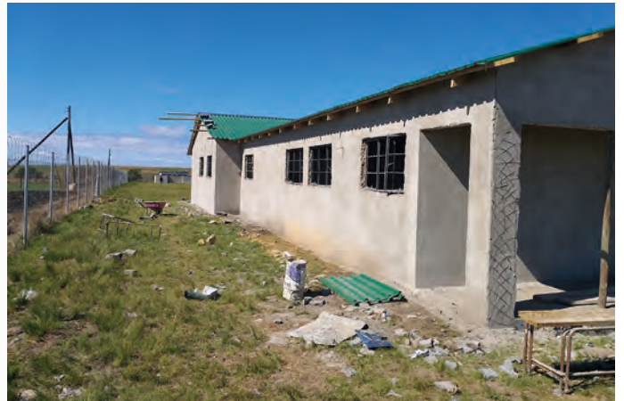
Building underway for foundation phase
